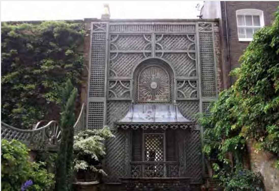
▲ ABOVE Tricoya Trompe- l'œil decorative feature finished with a shabby chic paint effect.
