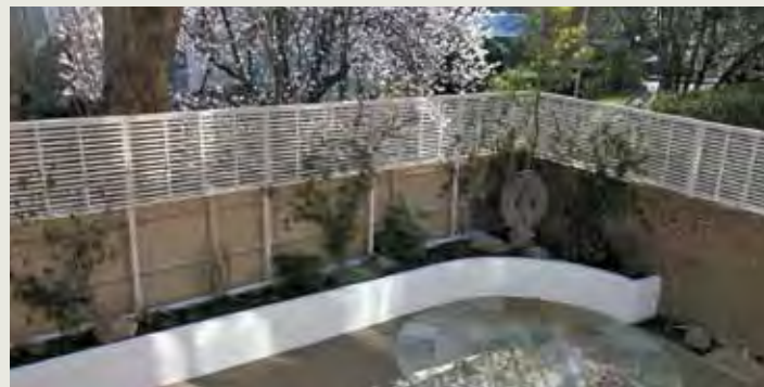
▶ RIGHT Bespoke slatted panels painted in Orford Cream, fitted on top of existing fencing and a boundary wall.
